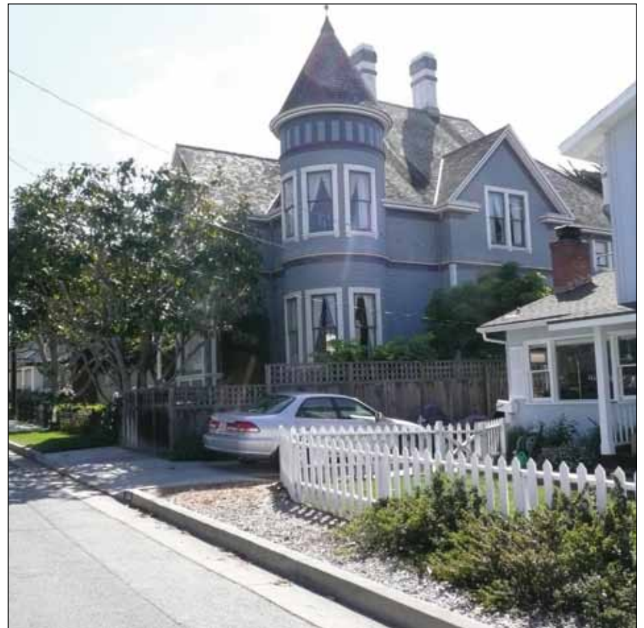
Above: Trimmer Hill is a historic home on 6th Street. Owners seek to add a garage to the rear of the building.
